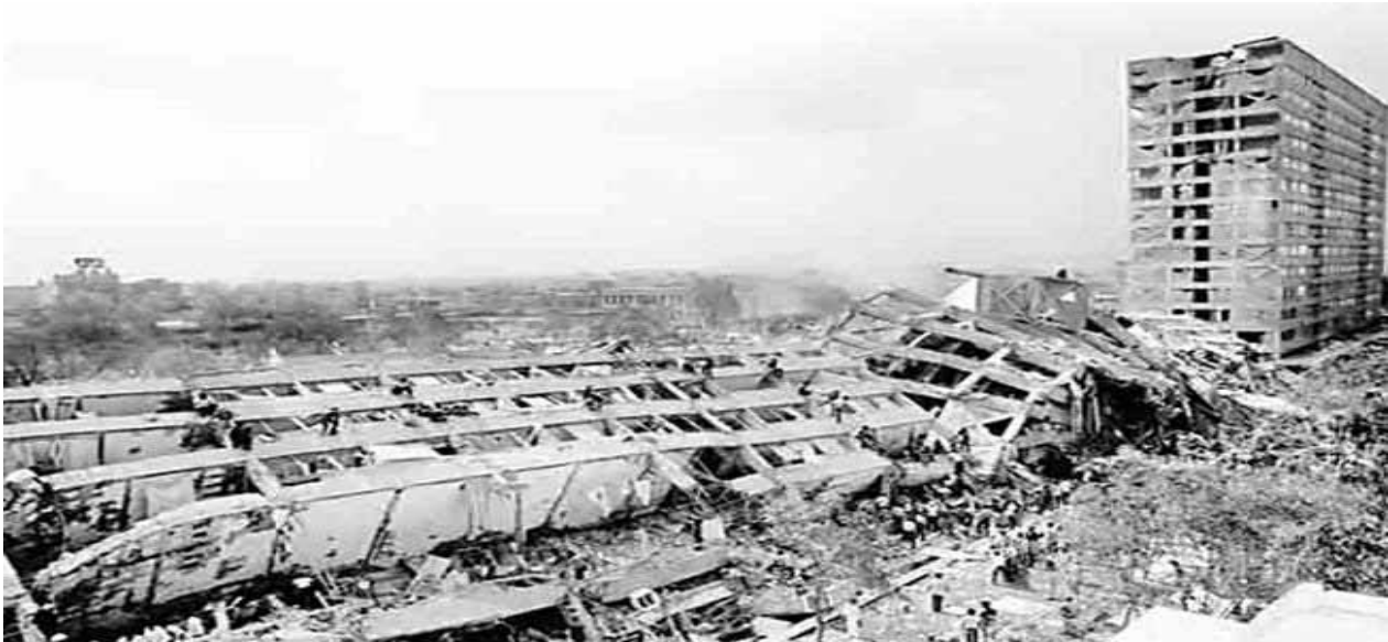
Pic.1 Damage buildings in Mexico City which is built on a sedimentary basin with a resonance frequency of about 1 Hz. Seismic Microzonation studies may be carried out at three levels:
